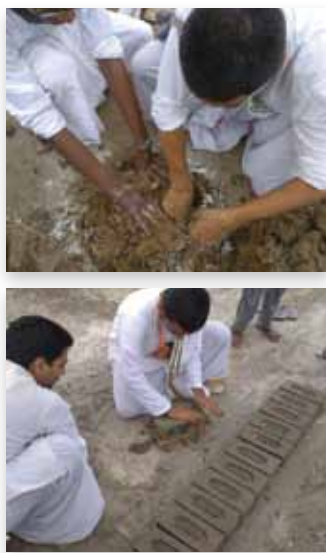
Fig 3,4 : Making mudbricks at site
